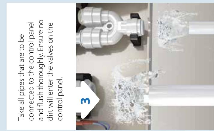
Take all pipes that are to be connected to the control panel and flush thoroughly. Ensure no dirt will enter the valves on the control panel.
