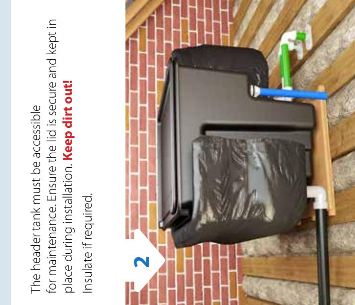
The header tank must be accessible for maintenance. Ensure the lid is secure and kept in place during installation. **Keep dirt out!**
