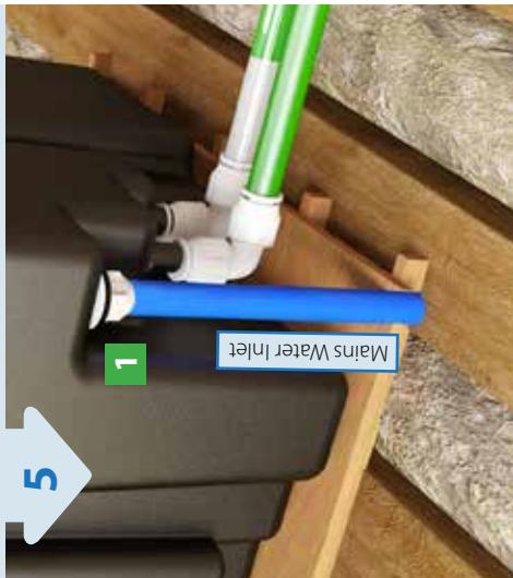
Fully fill the header tank and unscrew services cap. Wait for all air to leave the system to eliminate airlocks then replace cap ensuring that the black washer under the cap is replaced.
