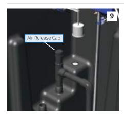
9) Fully fill the header tank and unscrew the air release cap. Wait for all air to leave the system to eliminate airlocks, then replace cap ensuring that the black washer under the cap is replaced.
