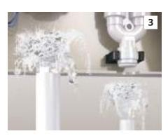
**3)** Take all pipes that are to be connected to the control panel and flush thoroughly. Ensure no dirt will enter the valves on the control panel.
