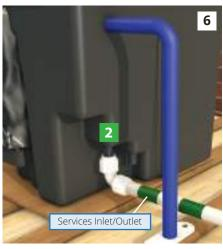
**6)** Connect the services feed from the control panel **(D)** to the header tank services inlet/outlet **(2)**.
