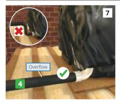
7) The overflow (4) must run straight out of the house without obstruction, bends, or decreasing pipe diameter. Use 40mm waste pipe elbow, either solvent or compression fitting.
