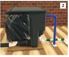
2) The header tank must be accessible for maintenance. Ensure the lid is secure and kept in place during installation. **Keep dirt out!** Insulate if required.
