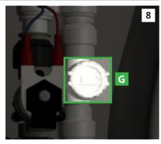
**8)** Use the quarter turn valve on the control panel **(G)** to partially fill the header tank.
