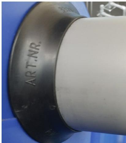
Feed a 4 inch pipe into the hole allowing at least 500mm to be inside the tank.
