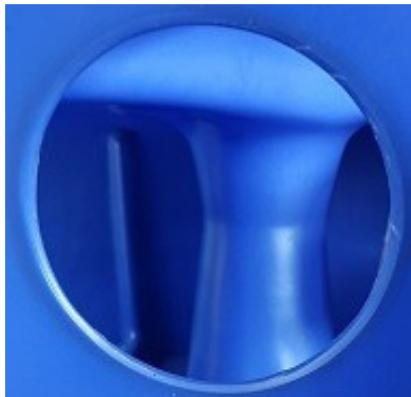
Drill a hole using a 127mm holesaw into a flat part of the tank at low level.
